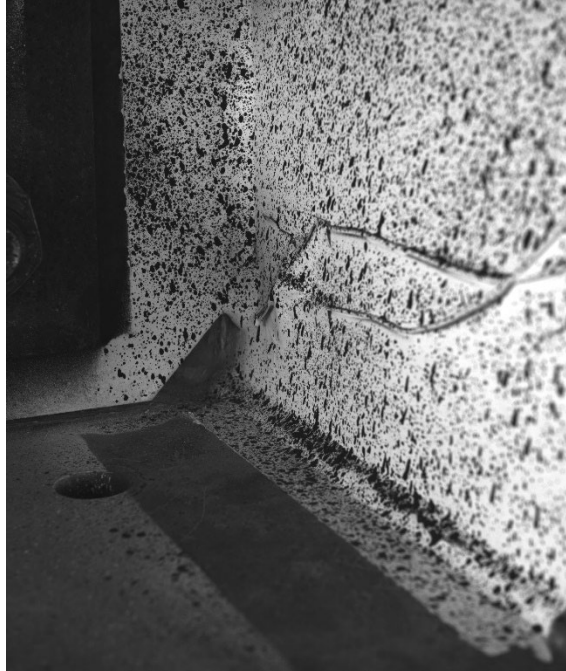
Figure B.10 Out-of-plane specimen under loading case 3
